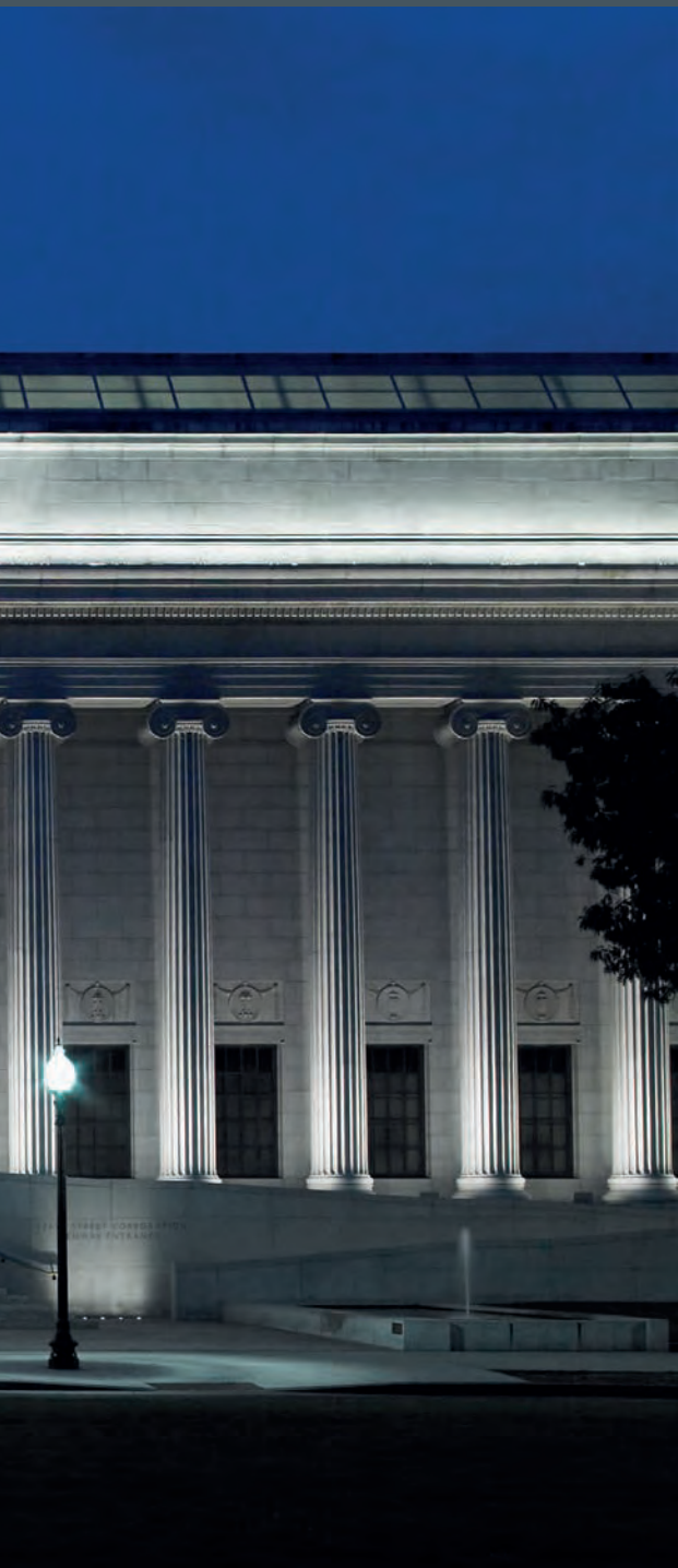
Lighting Design: George Sexton Associates, Washington, DC
