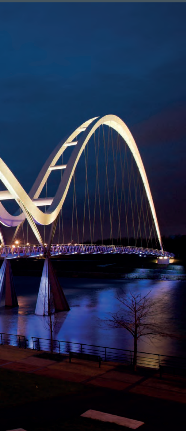
Lighting Design: Speirs+Major Associates, Edinburgh/London
